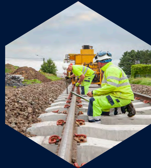
Mobility & energy infrastructure of tomorrow
